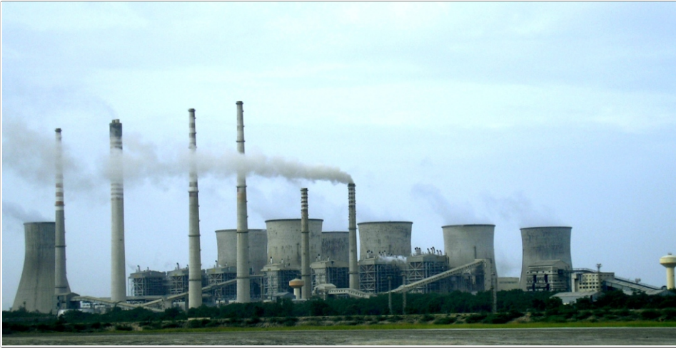
Raichur Thermal Power Station, Raichur
